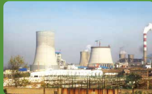
Shaanxi Qinling IDCT 2x600MW
