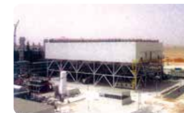
Hassi R'Mell Algeria ACC for 150MW combined Cycle Power Plant Solar Power Plant
