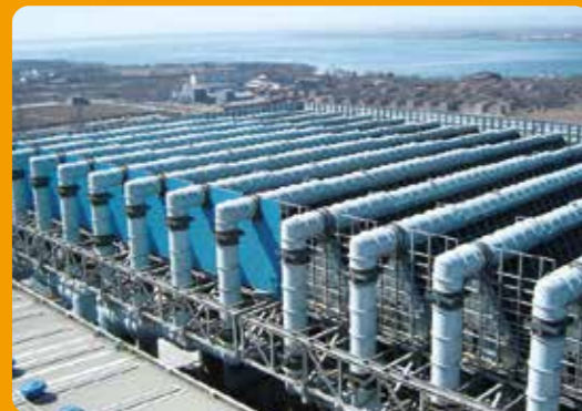
Mechanical Draft Air Cooled Condenser (ACC A-Frame)
