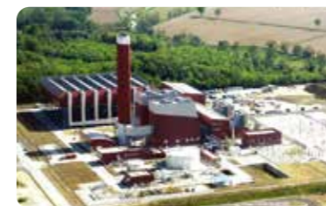
Turano Lodigiano Sorigenia 800MW combined Cycle Power Plant
